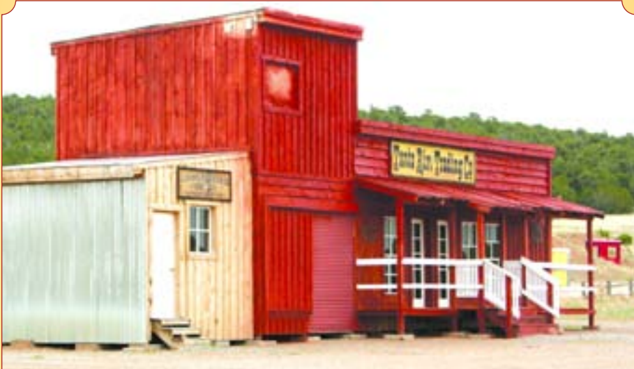
Eventually, all the mercantile buildings will be painted ... just like in the Old West!
