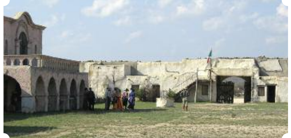
The interior courtyard of the fortress.
