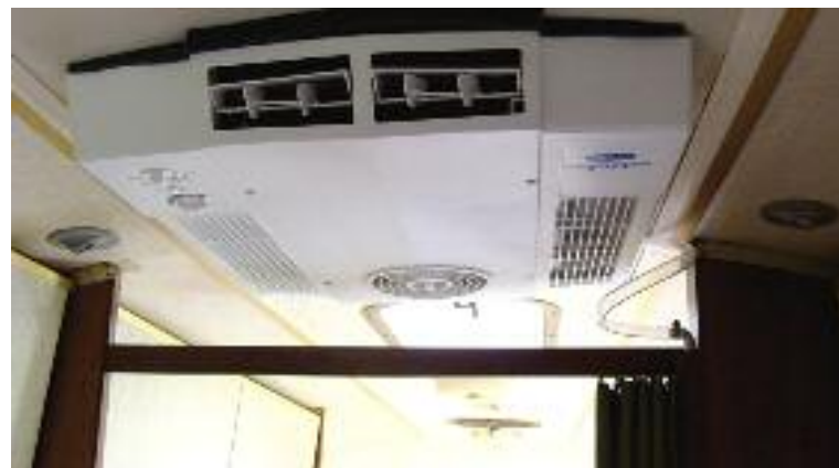
Ceiling unit shroud installed with drain line in place
