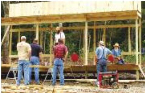
Rain slowed down the building of stages six through ten, but they were all finished before the match started.
