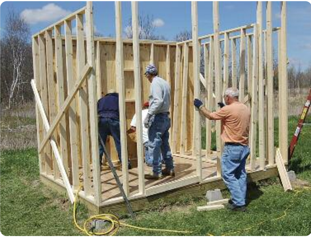
After the linoleum expanded somewhat, the 2" X 4" framed walls were set in place. The walls hold the linoleum in place.
