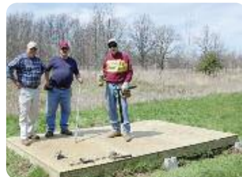
Treated 3/4" plywood covers the frame. This makes a very solid floor.
