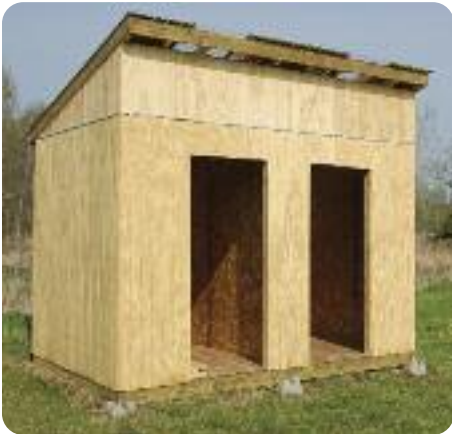
Outhouse roughed in. We used T-111 siding. Steel might be a little less costly.
