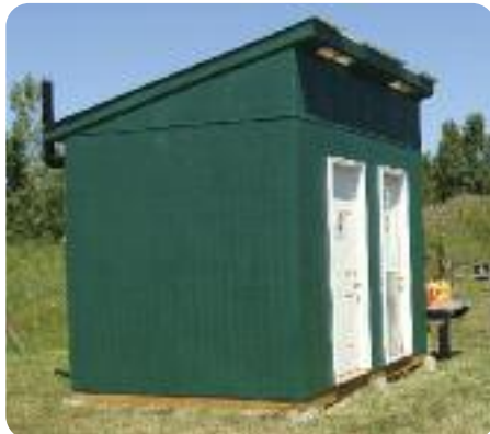
Finished outhouse painted dark green. The vent pipes are painted black so they heat up in the sun to help draw fumes better. Notice the screened in eaves over the doors. Between the vent pipes and the screened eaves, the outhouse is virtually odor free.
