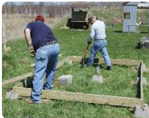
Leveling the outhouse deck. We set the 2" X 6" treated wood frame on concrete piers. It could just as well be set on crushed rock to let the water drain away.
