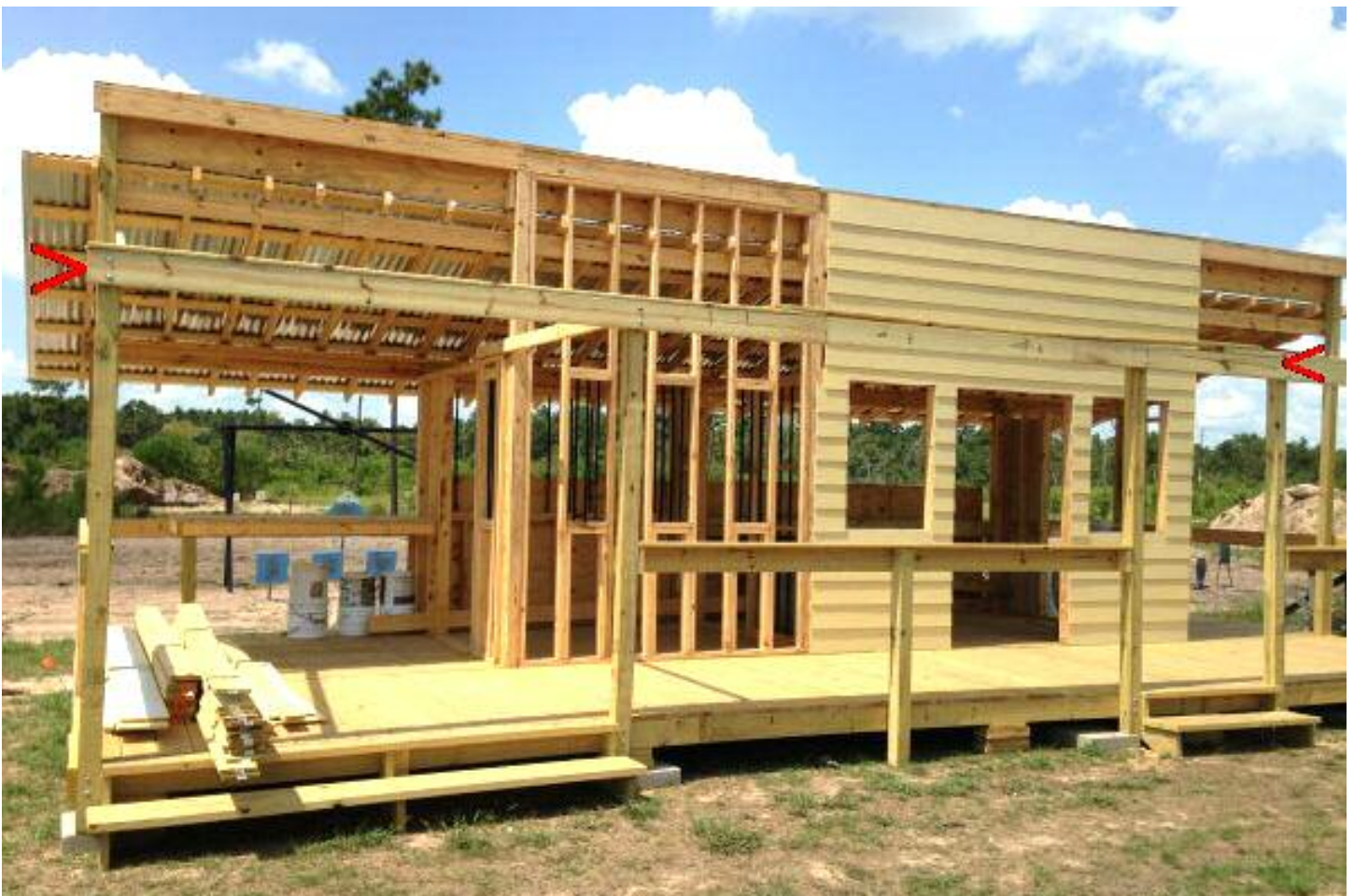
The new Tombstone Territorial Jail stage building under construction.
