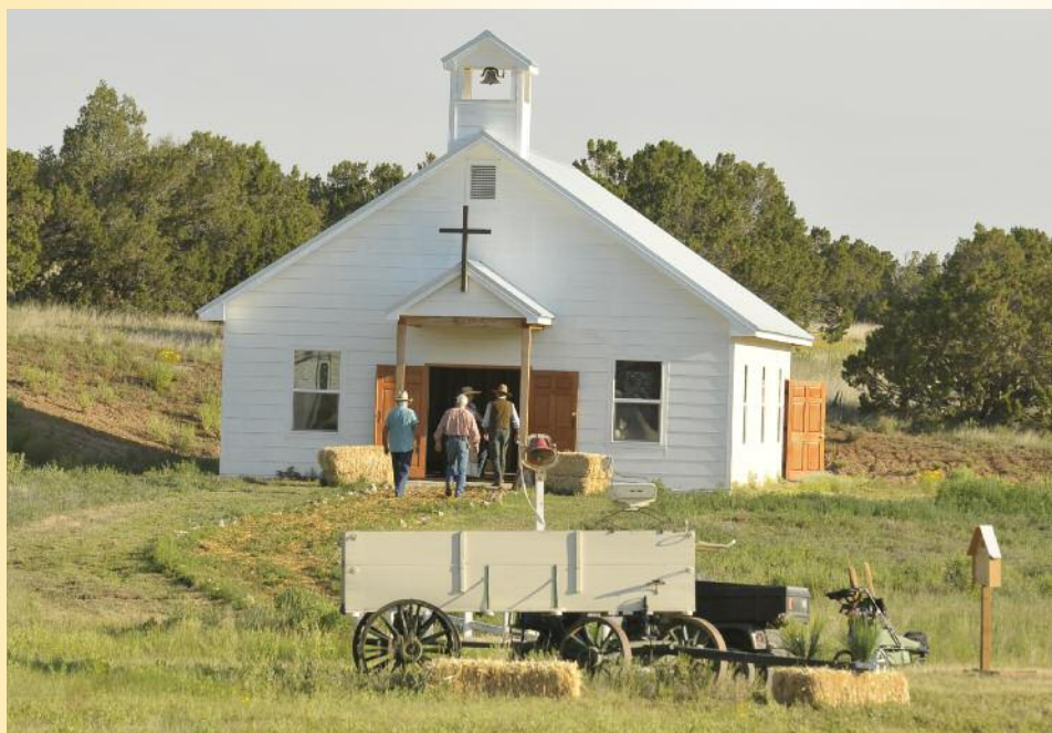
The Memorial Chapel continues to see double duty during END of TRAIL as a meeting hall and church. The Wild Bunch has made the commitment to finish what the Chapel Committee so ably got started... the interior will finally be completed by END of TRAIL 2016! The Chapel is in place because of the efforts of the Chapel Committee—Thank You!
