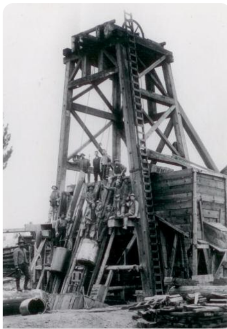
Steel drums were used to haul up rock, debris, and water that seeped into the shaft.
