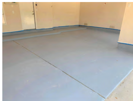
AFTER EPOXY PAINTING THE GARAGE FLOOR.
