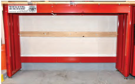
A 2 X 4 WAS ATTACHED TO THE STUDS THEN THE WORKBENCHES WERE LEVELED AND ATTACHED TO THE 2 X 4S.
