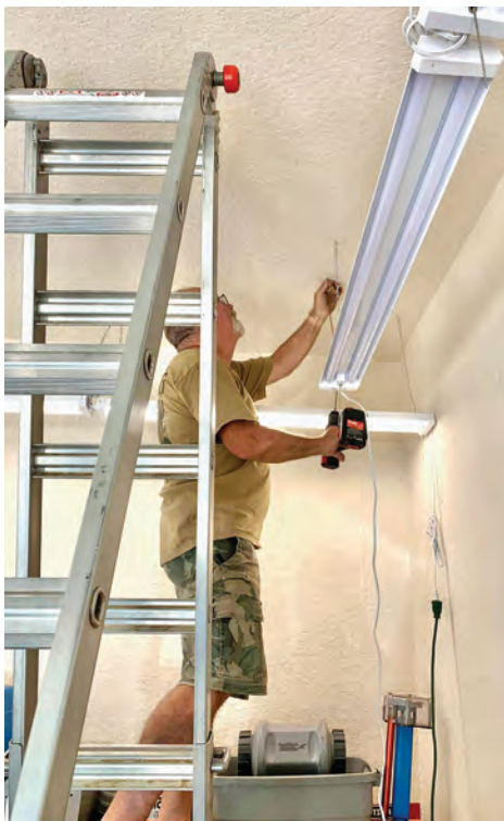
DAWGTOOTH DAVE INSTALLED SIX DOUBLE LED FOUR-FOOT LIGHT UNITS. THEY WERE LINKED TOGETHER AND ARE CONTROLLED BY THE LIGHT SWITCH. THE WIRING IS TO CODE.
